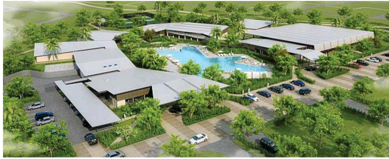
RESORT LIVING: Recreational facilities are the resort will include a lagoon pool, cinema, games room and tennis courts.
